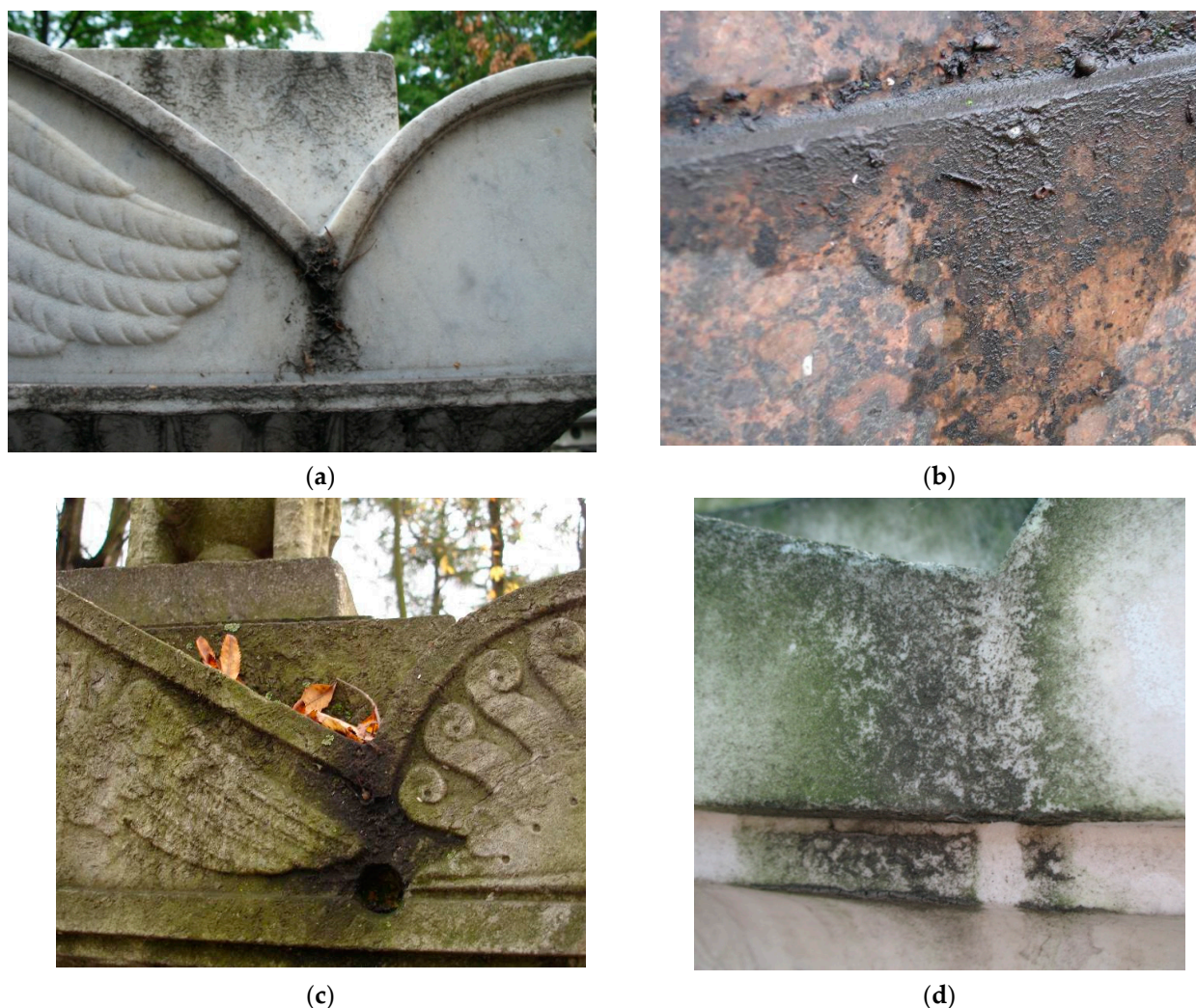
Figure 1. Superficial deposits on the surface of the monuments of the Historical Necropolises in Saint Petersburg: (a) Superficial deposits on marble monument; (b) superficial deposits on granite monument; (c) superficial deposits, leaf litter, and biofilms formation on the monument; (d) Algae biofilm growth on superficial deposits.
