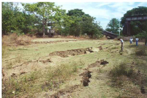
Fig. 20 Lateral spreading on the bank of the Lempa River in El Salvador due to liquefaction triggered by the M 7.7 subduction-zone earthquake of January 2001; notice the collapsed railway bridge in the background due to the separation of the piers caused by the spreading (Bommer et al. 2002)
