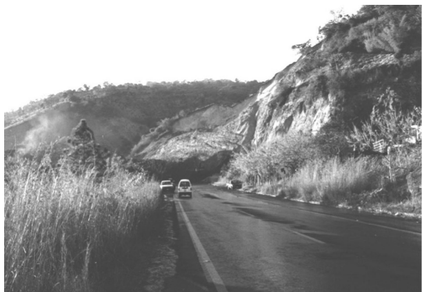
Fig. 19 Major landslide triggered by the El Salvador earthquake of January 2001 (Bommer and Rodriguez 2002); another landslide triggered in Las Colinas by this earthquake killed around 500 people
