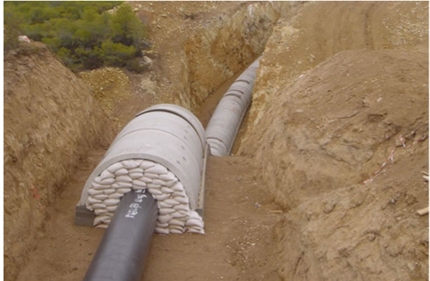
Fig. 11 Construction of high pressure gas pipeline from Megara to Corinth, Greece: where the pipeline crosses active faults, it is encased to prevent damage due to fault slip (Image courtesy of Professor George Bouckovalas, NTUA http://users.ntua.gr/gbouck/proj-photos/megara.html )
