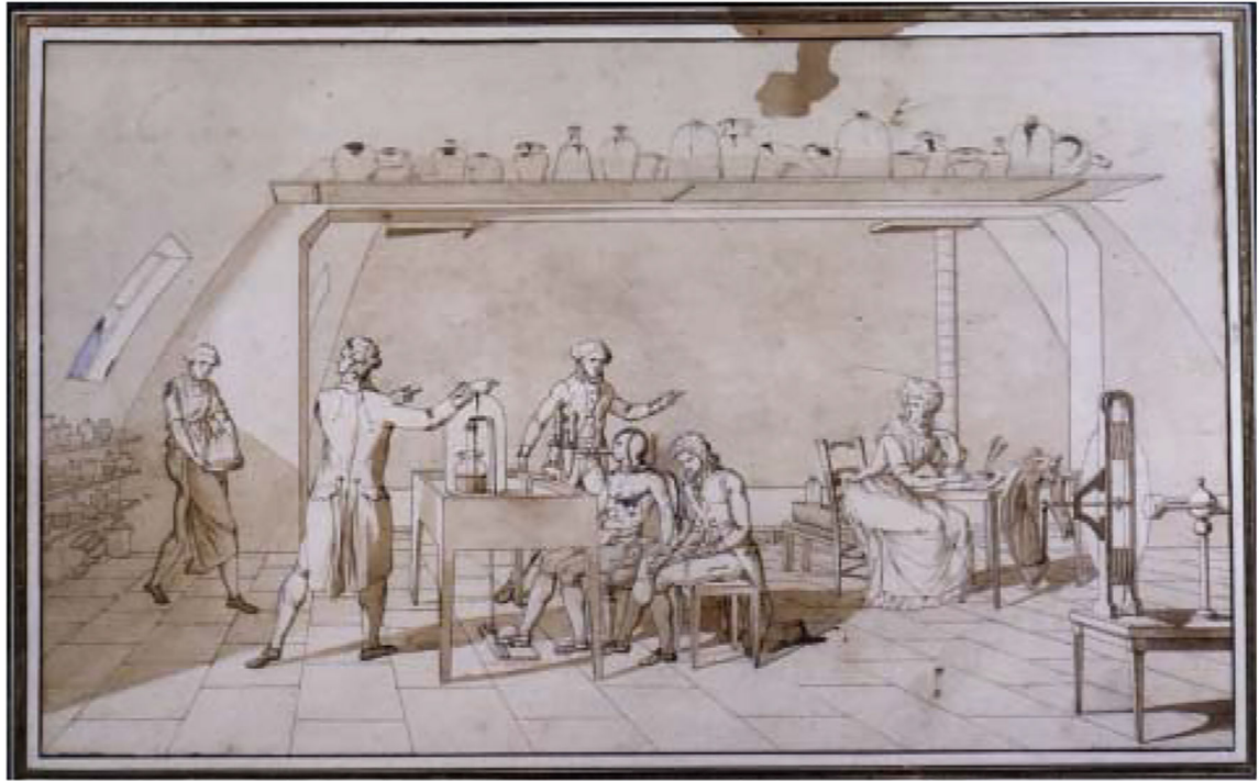
Figure 1. Marie-Ann Pierrette Lavoisier's sketch depicting her husband Antoine Lavoisier conducting the first exercise physiology experiment and herself taking notes in the right corner. Note the use of the bell-jar calorimeter and the subject pressing a foot pedal below the table. Reused, with permission, from West JB, 2013 (1416).
