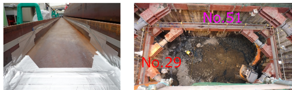
Figure 14. Displacement measurements, installed fiber (left), and construction site (right).
