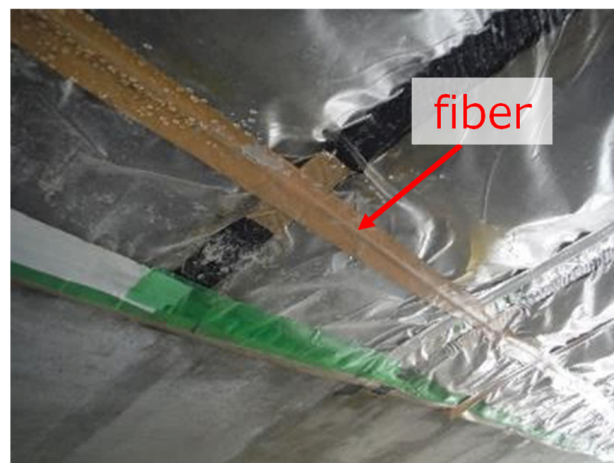
Figure 25. Fiber installation.
