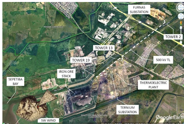
Figure 5. The transmission line and the three towers, with the sensors installed. The transmission line transports the energy generated by the Ternium Steel Co. thermoelectric plant to the Furnas National Grid Substation.
