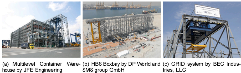
Fig. 7. Prototypes of new terminal system. (a) Multilevel Container Warehouse by JFE Engineering, (b) HBS Boxbay by DP World and SMS group GmbH, (c) GRID system by BEC Industries, LLC.
