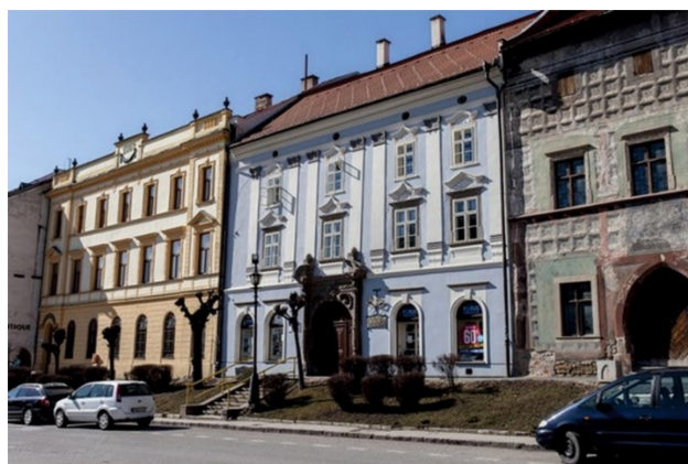
Figure 4. Current state of building no. 43 in Master Paul’s Square, view from the square.
