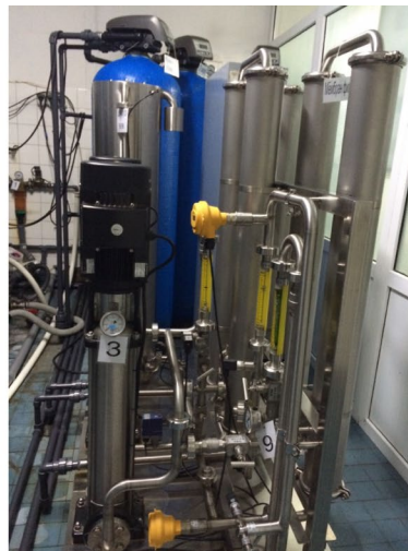
Fig. 11 The scene of Dialysis Center at First Central Hospital of Mongolia. The storage tanks for dialysis water were a suitably small size for dialysate purification
