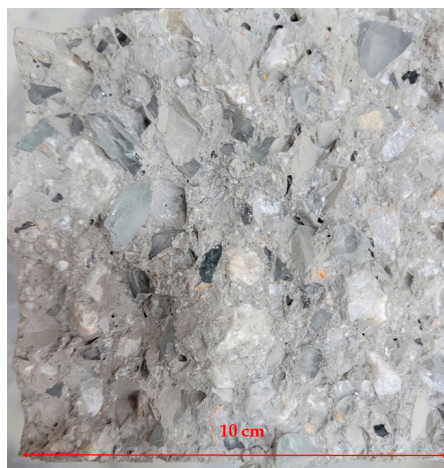
Figure 2. Recycled glass in concrete.
