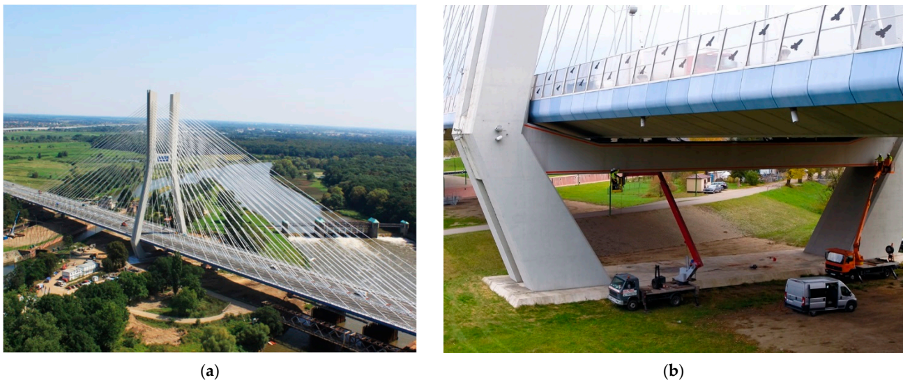
Figure 19. (a) Rędziński Bridge in Wrocław, Poland—general view (photo: W. Kluczewski); (b) the close-up of the lower crossbeam connecting two inclined legs of the pylon.
