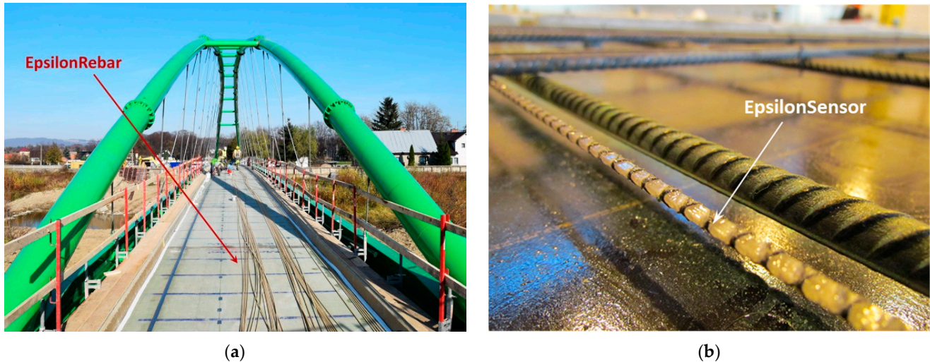
Figure 6. (a) Footbridge reinforced with stiff monolithic sensors; (b) concrete slab with the flexible monolithic sensor not influencing the structural behaviour [8].
