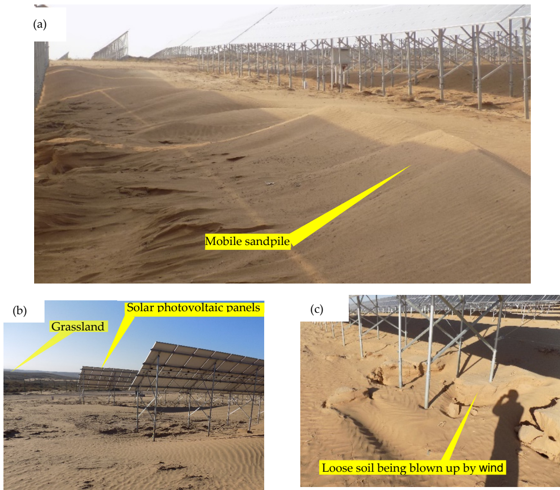
Figure 2. An onsite view of 25 October 2016, land desertification caused by the photovoltaic power generation project in Zhongning County, Ningxia Province. (a) Mobile dunes had been formed in the constructive area. (b) The land in the construction area was undergoing desertification, and the land outside the construction area was still grassland. (c) The soil around the support of the photovoltaic panel was blown away by the wind.
