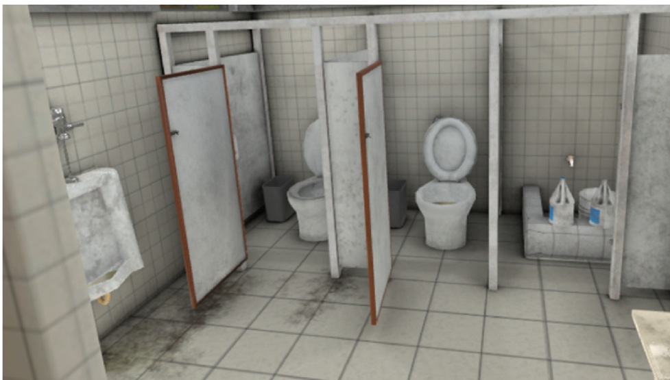
Figure 7. Level 1 of dirtiness in bathroom.
