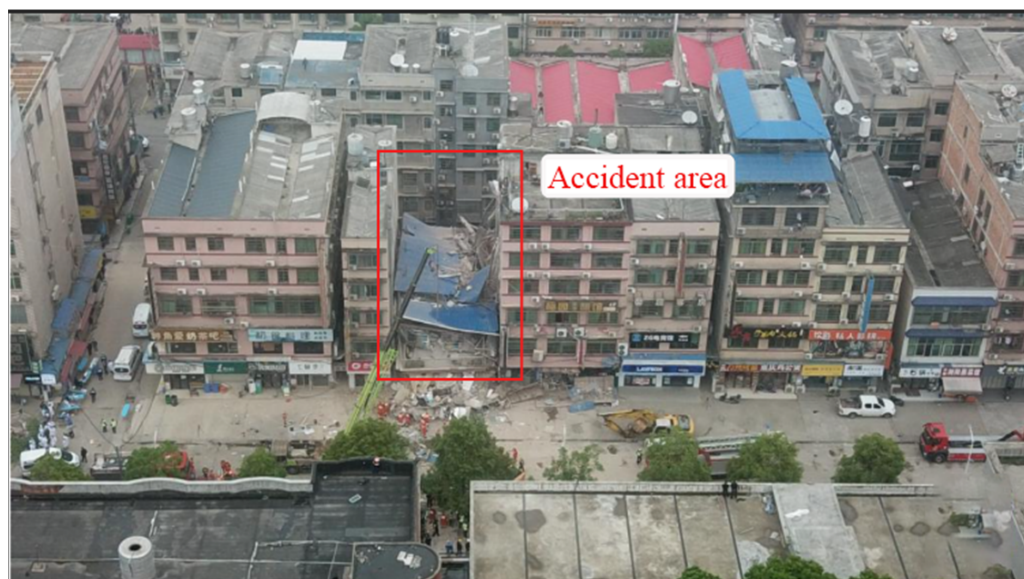
Figure 3. Photo of the collapse site.
