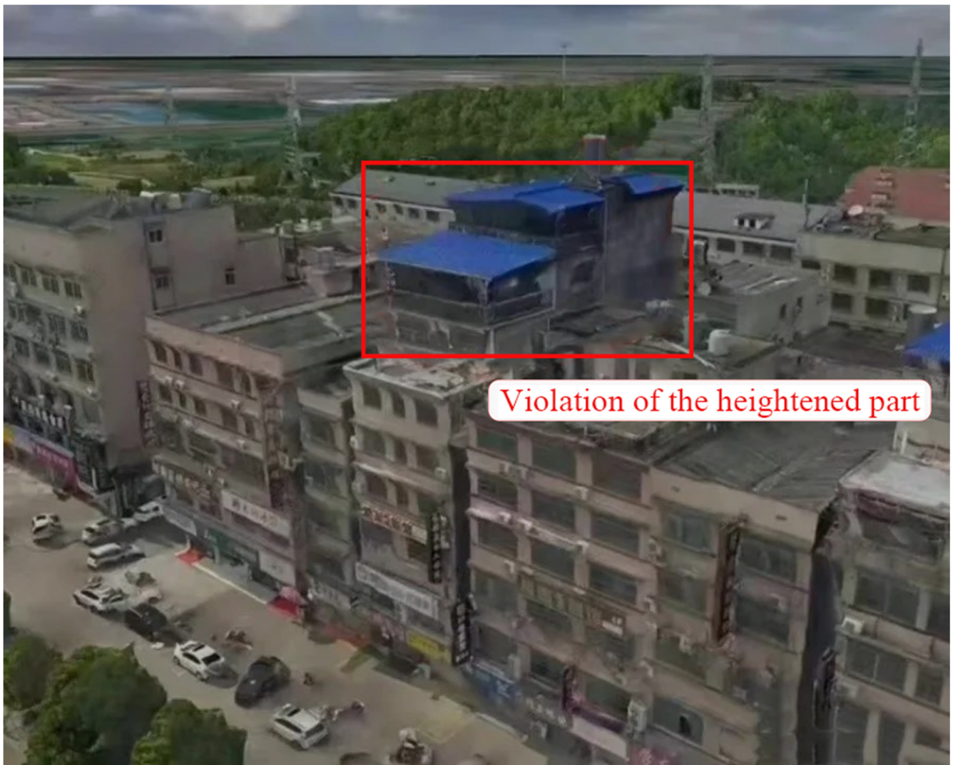
Figure 5. Collapsed building original structure.
