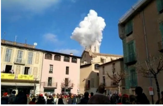
Figure 1. The bell tower seconds after the explosion (retrieved from Twitter with permission from the author).
