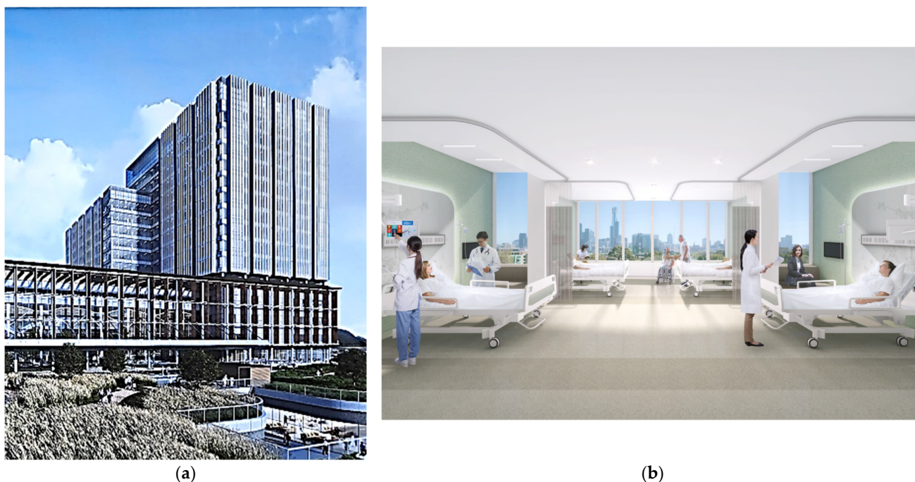
Figure 5. (a) The lower section of the hospital includes an outpatient department, central medical labs, and administrative department. The upper tower is dedicated to an inpatient department. Unlike the typical hospitals, the overall shape of the tower is not linear but rectangular to enhance the daylight condition in the inpatient wards and to reduce the corridor length traveled by nursing staff; (b) The design of the four-person inpatient unit type is devised to improve the daylight, view, and privacy for each patient by an extensive exterior glazed window, an alcove-shaped room, and bed arrangement. (Source: (a) photo by author taken from the construction site, (b) image from Samoo Architects & Engineers; The original competition-winning design was proposed by Samoo Architects & Engineers).
