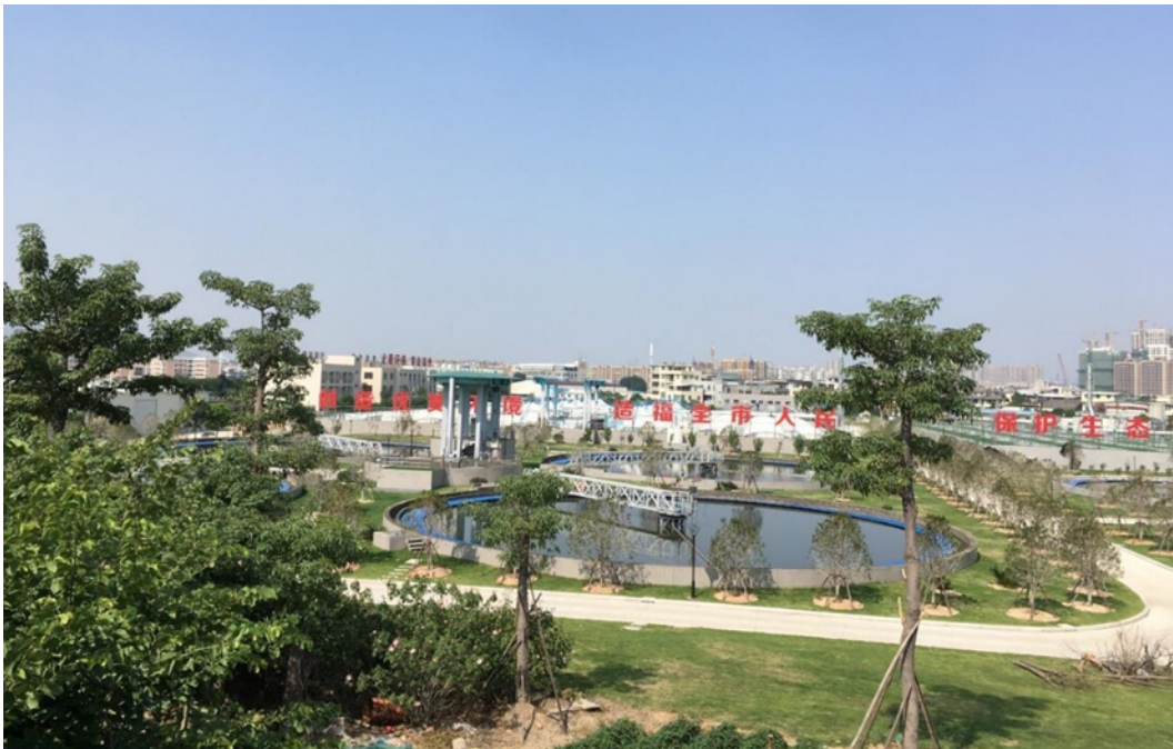
Fig. 2. The Sewage Treatment Plant (Plant B) in Fuzhou, Fujian Province, China, was Used as the Case Study to Test the Proposed Performance Evaluation System
