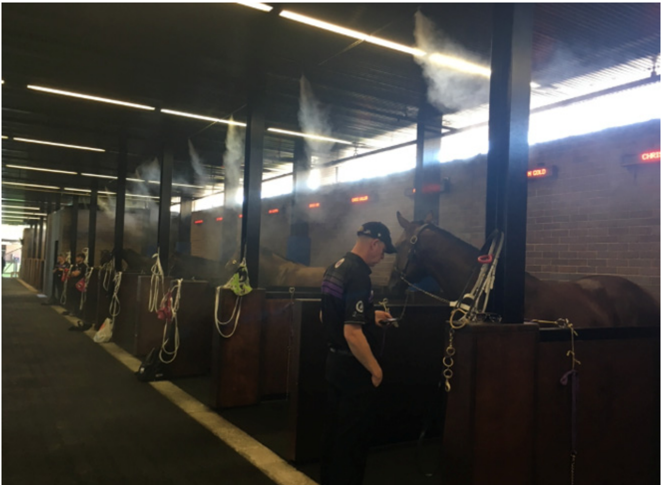
Figure 27. Misting sprays in the tie-up stalls at a racecourse in Australia. The devices can theoretically increase the humidity by up to 20% in the immediate vicinity, negatively affecting thermoregulatory capacity.
