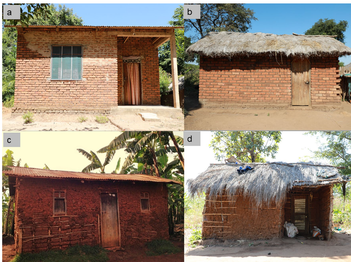
Fig. 2 Common house types in the study sites: a brick walls with metal roof, b brick walls with thatched roof, c mud walls with metal roof, d mud walls with thatched roof
