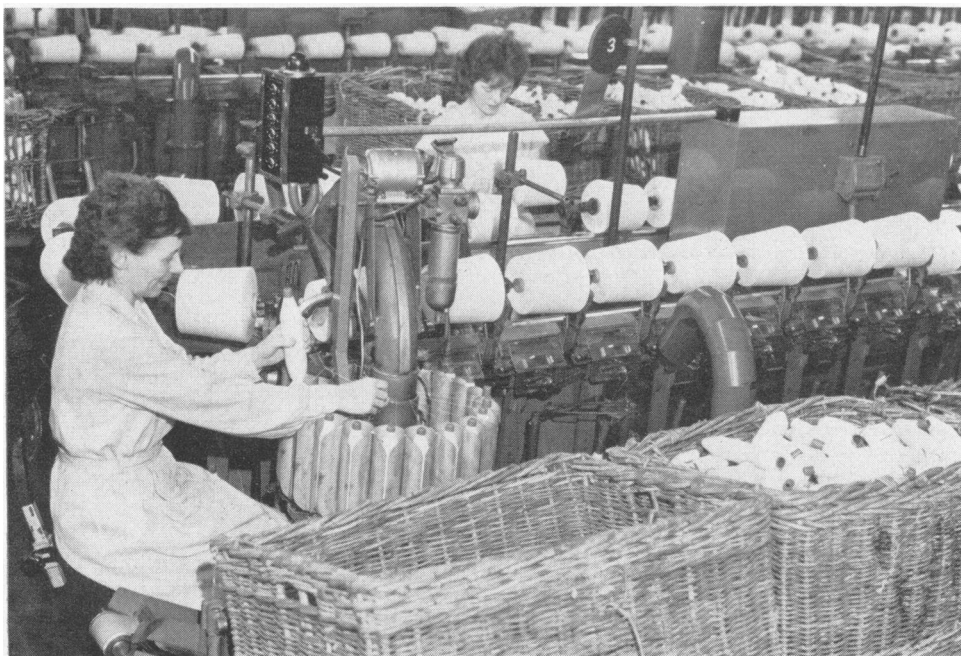
FIG. 1. Abbott winding.
