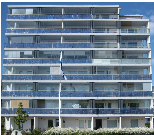
Figure 1 Solar panels, integrated in a block of flats in the Latokartano ecological housing area (Helsinki, Finland). https://upload.wikimedia.org/wikipedia/commons/6/66/Solar_panels_integrated_in_a_block_of_flats_in_Viikki_Helsinki_Finland.jpg Credit: Pöllö.
