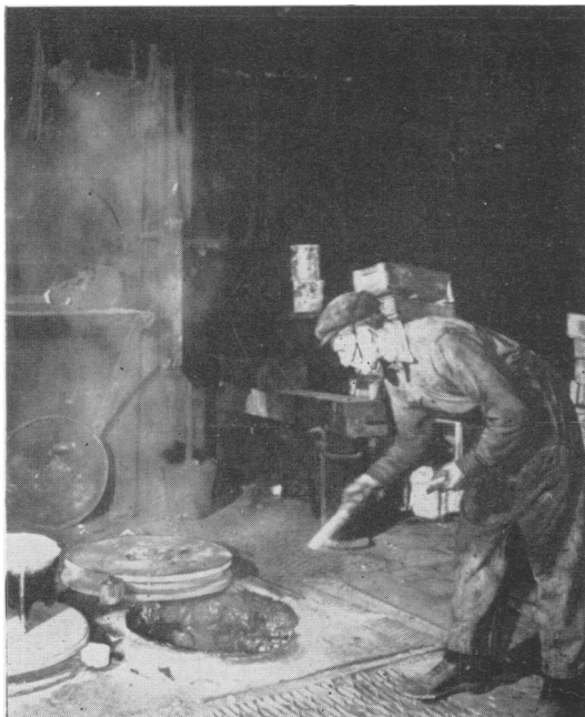
FIG. 2.—Oil-fired pit-fire furnace in factory B.
