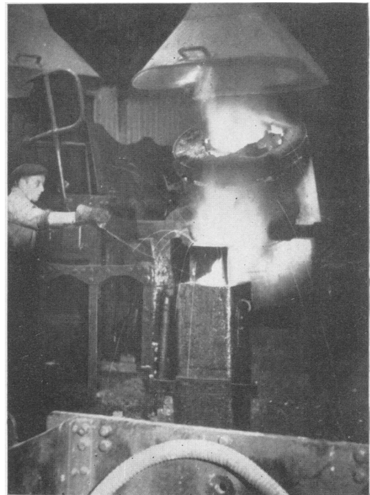
FIG. 3.—Oil-fired tilting furnace in factory B.
