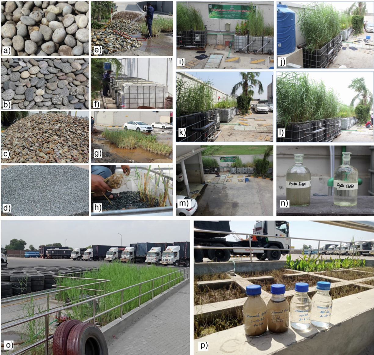
Fig. S5. Development of integrated system for the treatment and reuse of vehicle-wash wastewater at Toyota Lyallpur Motors Faisalabad, related to STAR Methods. Gravel at the bottom of the tank (a), second layer of the gravel (b), third layer of the gravel (c), and fourth layer of the gravel (d), washing of the gravel (e), twenty tanks in the series (f), seedlings of the plants (g), and vegetation of seedlings in the gravel (h). Installation of automatic integrated system at Toyota Lyallpur Motors, Faisalabad (i-m) for the treatment and reuse of car-wash wastewater, the water in the reagent bottles (n) shows the water collected at inlet and outlet. Development of integrated system of floating treatment wetlands, constructed wetlands and sand filtration at Interloop Logistics Momentum Khanewal (o) for the treatment and reuse of containers-wash station. The bottles shown in (p) contain water collected at the inlet and outlet.
