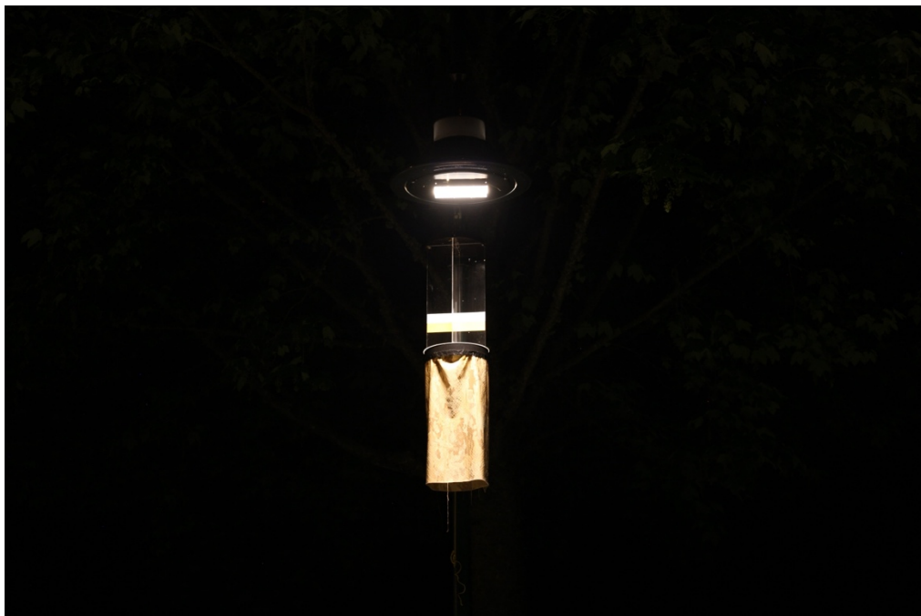
Supplementary Figure 14: Road lights at the Municipal Site Heimbachau. Photos were taken from the same distance to luminaire. Conventional luminaires (HPS bow-shaped, E_m = 5.1 lx, CCT 2000K) (top) and tailored and shielded luminaires (LED, E_m = 5.1 lx, CCT 2700K) (bottom). n=7 samplings, 4 luminaires per treatment.
