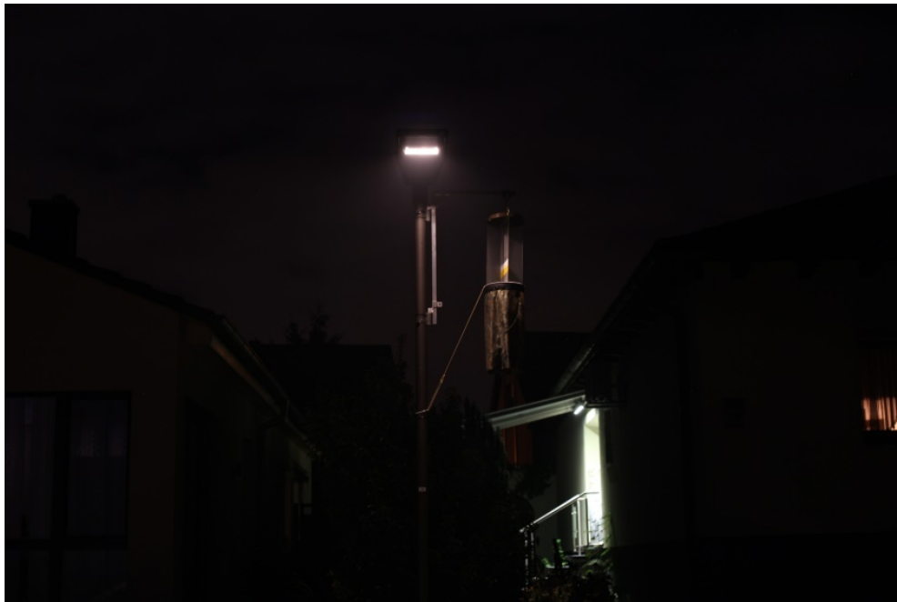
Supplementary Figure 11: Road lights at the Municipal Site Backofen Riedwiesen. Photos were taken from the same distance to luminaires. Conventional luminaires (HPS cylinder, E_m = 3.1 lx, CCT 2000K) (top) and tailored and shielded LED luminaires ( E_m = 3.1 lx, CCT 2700K) (bottom). n=7 samplings, 5 luminaires per treatment.
