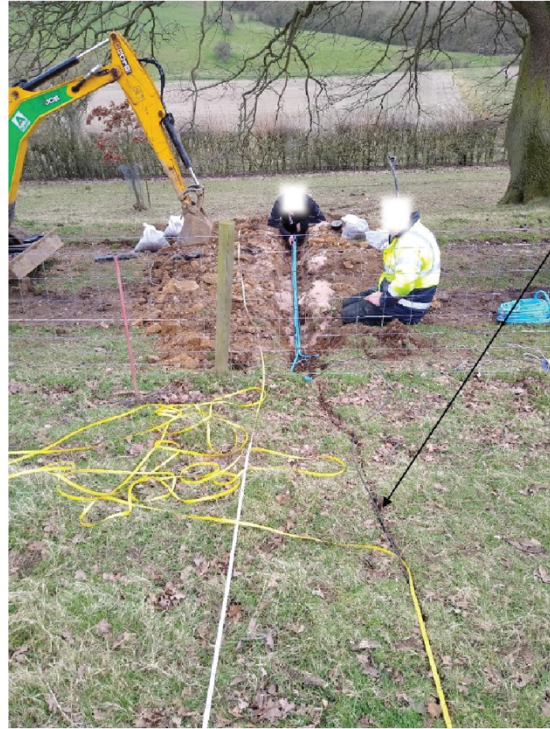
Fig. S1 Photos of the fiber optic installation, showing the transition from protective housing to the bare cable at Hollin Hill. Faces have been blurred to conceal identities of individuals in photograph.
