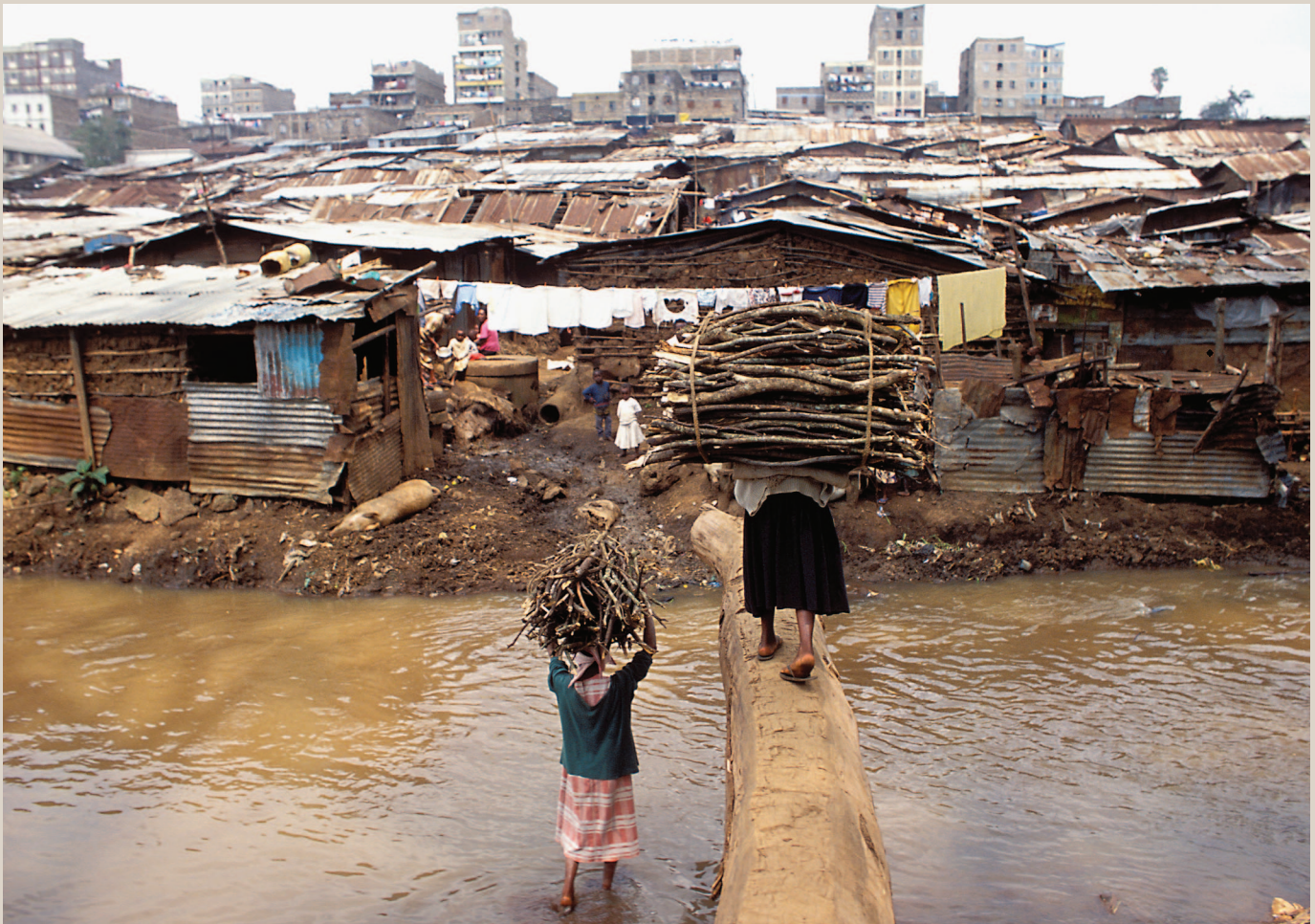
Bleak prognosis. Overcrowding, poor indoor air quality from the use of biofuels, and lack of clean water and sanitation—all apparent in this slum in Nairobi, Kenya—are only a few of the many housing-related deficiencies that can lead to serious health problems.
