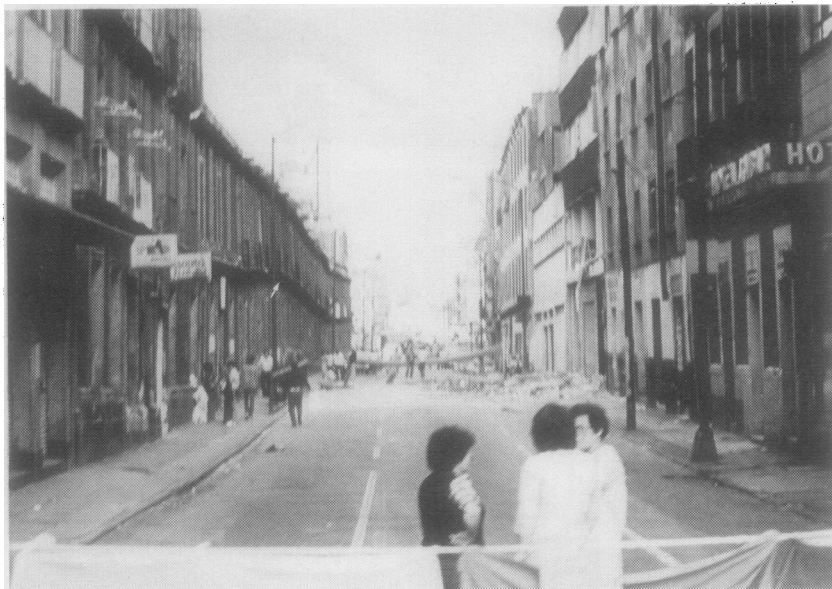
The white arrow on the left third of the photo points to a "wave" in building created by the earthquake.
