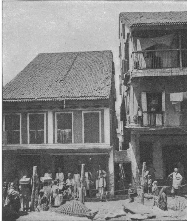
Bombay City: showing country tiles on roofs and a gully between the houses.
