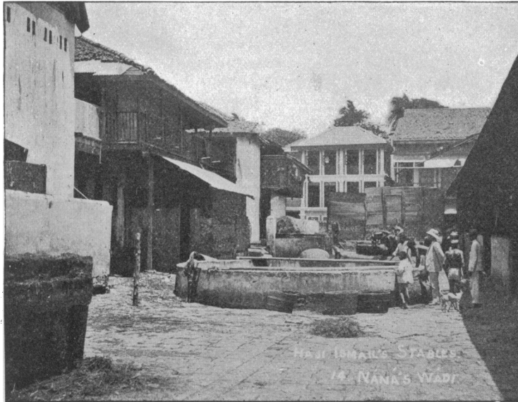
Bombay City: showing Courtyard with stables.
