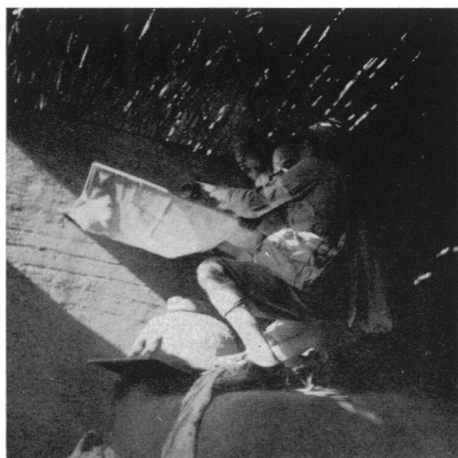
FIG. 25. DISINSECTIZATION OF AUTOMOBILES. The car is covered with a large sheet held close to the car, while the mulahez sprays the insecticide. After spraying, the sheet is retained for 5 minutes.
