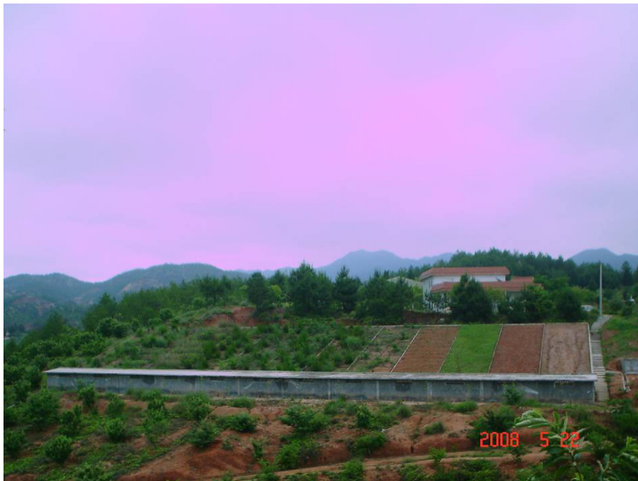
Fig. S7. To monitor run-off and soil erosion in Changting County, sedimentation ponds were constructed on representative slopes at each village ( Top ) and artificial sand sedimentation ponds ( Bottom ) were constructed at a monitoring station used for the soil and water conservation project.
