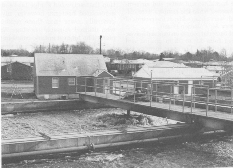
FIG. 1. Small activated sludge plant in a subdivision in Jefferson County, Ky., showing the proximity of aerated sludge to residences.
