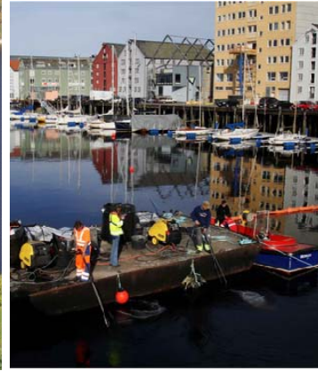
c) Application of activated carbon slurry directly onto sediments at Trondheim Harbor, Norway (2007). AC-salt water slurries with/without powdered bentonite clay were pumped 3-5 ft above the sediment bed under 20 ft of water. Part of the AC-only field was successfully covered with 5 mm sand to protect from erosion.
