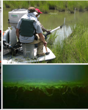
d) Application of activated carbon in a pelletized form (SediMite™) using an air blown dispersal device over a vegetated wetland impacted with PCBs near James River, VA, USA (2009). Picture below illustrates bioturbation induced breakdown and mixing of pelletized carbon with a fluorescent tag in a laboratory aquarium.
