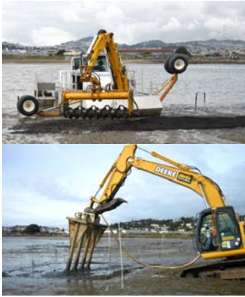
a) Application of activated carbon in a tidal mud-flat at Hunters Point Navy Shipyard, San Francisco Bay, CA using two application devices (2004 and 2006). The Aquamog (top) using a floating platform approached the site from water and used a rototiller arm while the slurry injection system (bottom) was land based and applied a carbon slurry directly into sediment.
