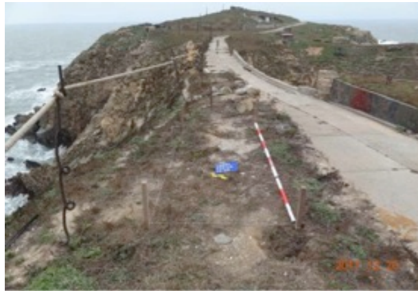
(b) LDDW-I site, the surface conditions prior to excavation, in the area within wooden poles; the road (right) is at a lower level
