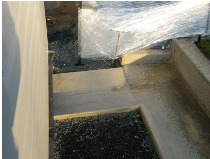
Figure S1-3. Movement from curb to flow and sampling equipment.
