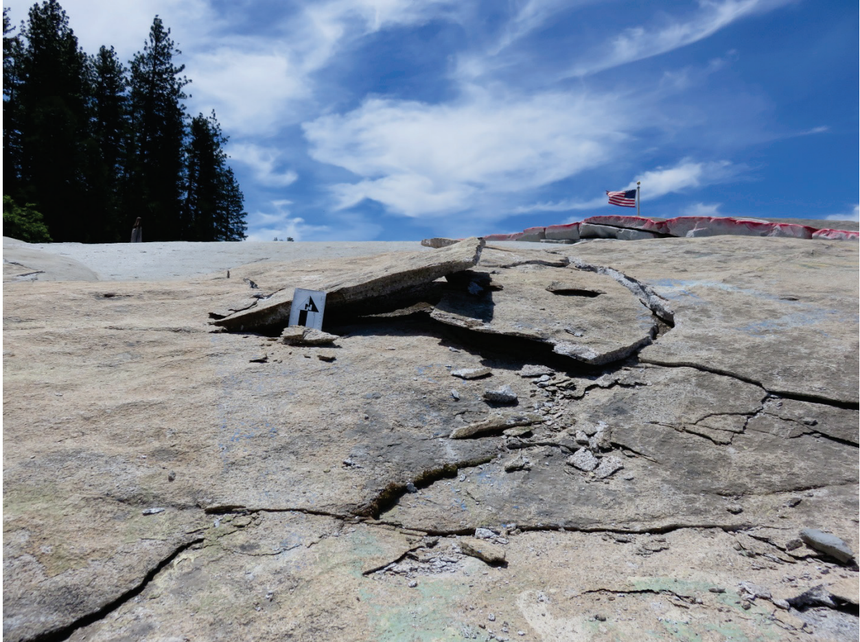
Supplementary Figure 1. Tent structure formed by energetic exfoliation fracture on 7 June 2016 at Twain Harte Dome. Total fracture occurred over a 15.6 m 2 area with 25 cm uplift of a 10 cm thick granodiorite exfoliation sheet. The event thrust rock fragments and dust 2 m in the air and was preceded by several minutes of audible cracking sounds. Scale bar is 15 cm. Several-millimeter-thick deposit of dark brown soil is visible to the right of the scale bar and under the tilted rock sheet indicating that the sheet was partially detached for some time prior to rupture. Exposed exfoliation sheets from energetic events in 2014 are visible in the background beneath the flag.
