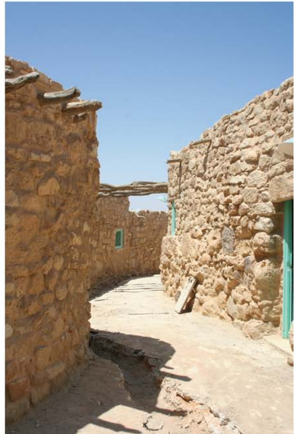
Fig. S20. Photos, taken in 2011, showing some examples of Juniperus phoenicea timbers in use in doors, doorways, roof/ceiling beams and other structural elements at Taybet Zaman.
