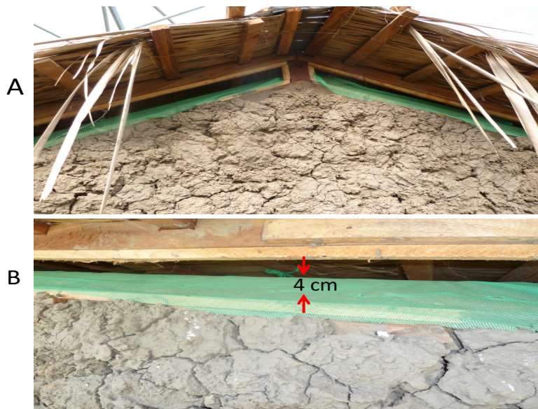
Figure S1: Photograph showing (a) eave louvers installed on the eave of the human hut in the mesocosm (b) close look of the gap and the netting material embedded on the wooden surface of the eave.
