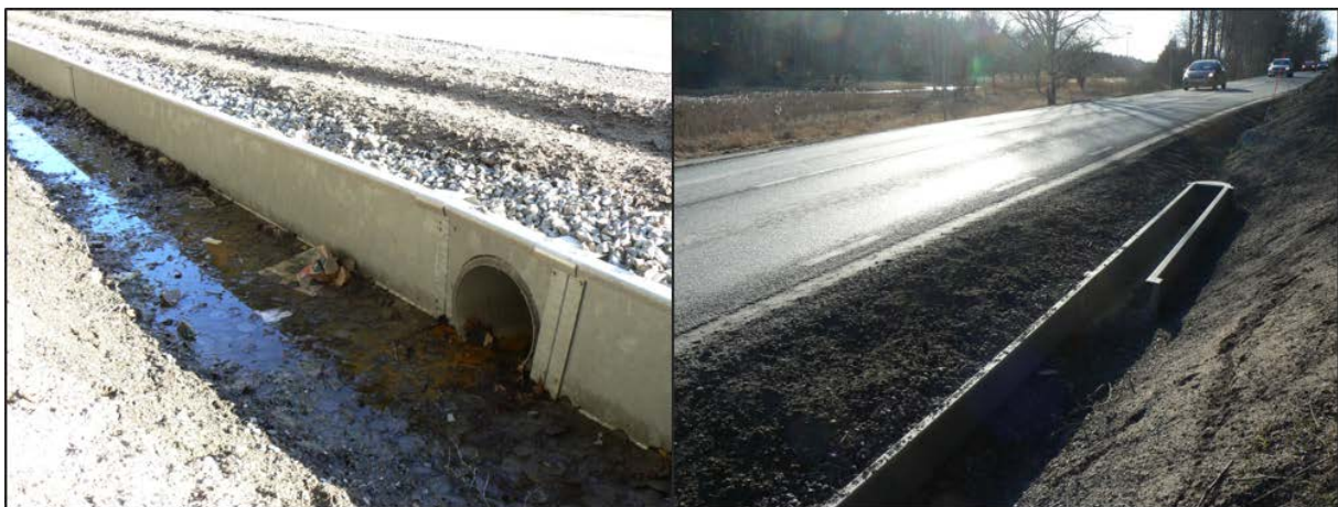
Figure S7. Amphibian tunnel, fence and fence-end at Skeppdalsström, Sweden. Photo: Jan Olof Helldin
