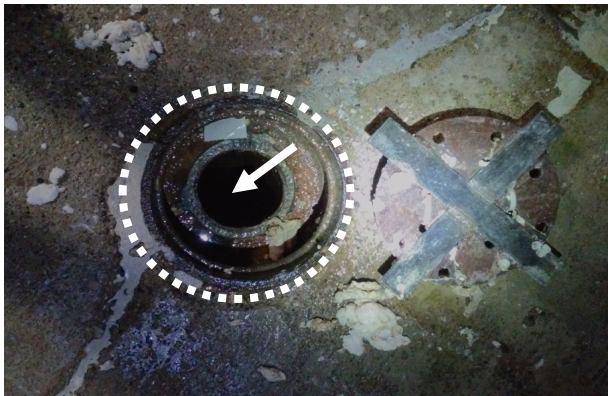
B. Standard industrial drain with top grate removed (A8, A9).
