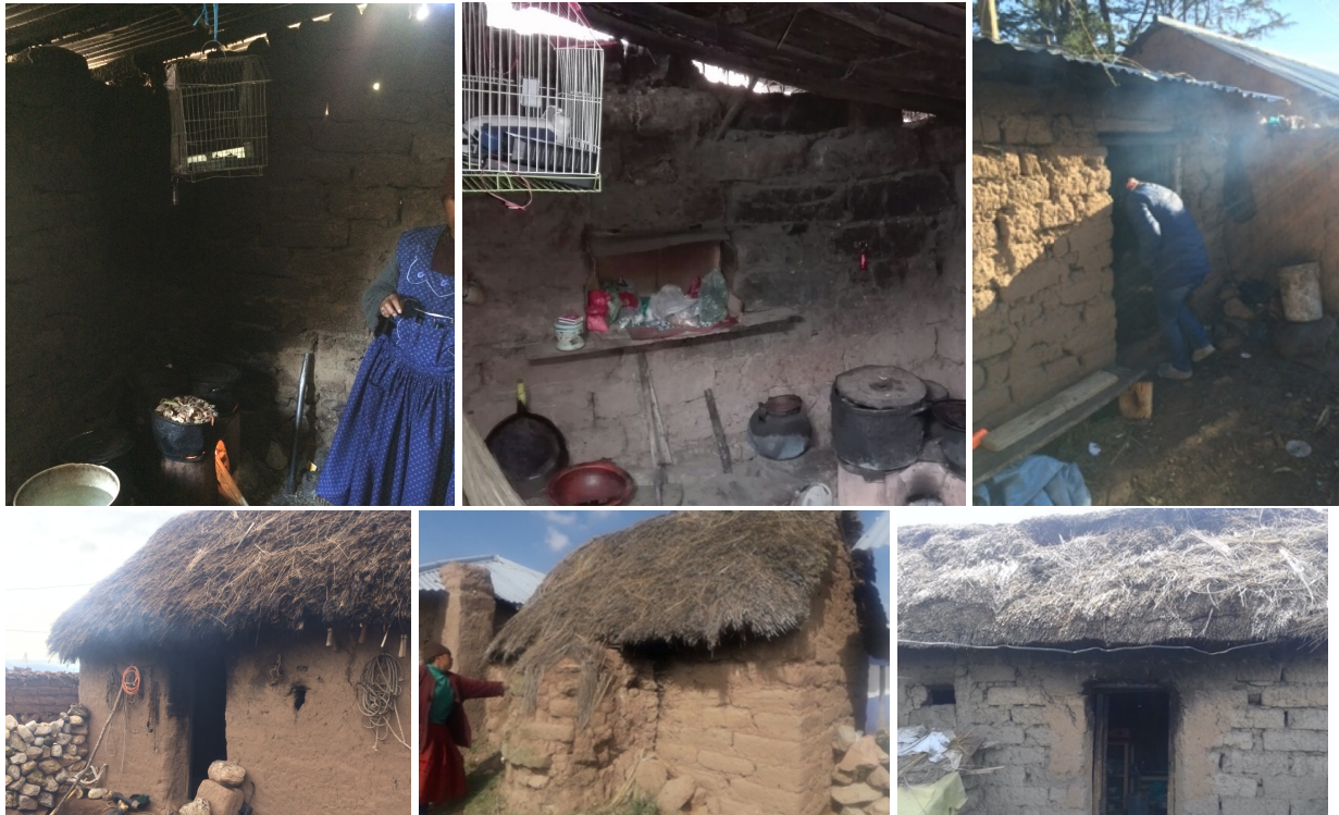
Figure S1. Metal roofs and natural material roof pictures of kitchen households from participants. Top pictures: metal roofs highlighting the space from the eaves; bottom pictures: kitchens with natural roof materials.
