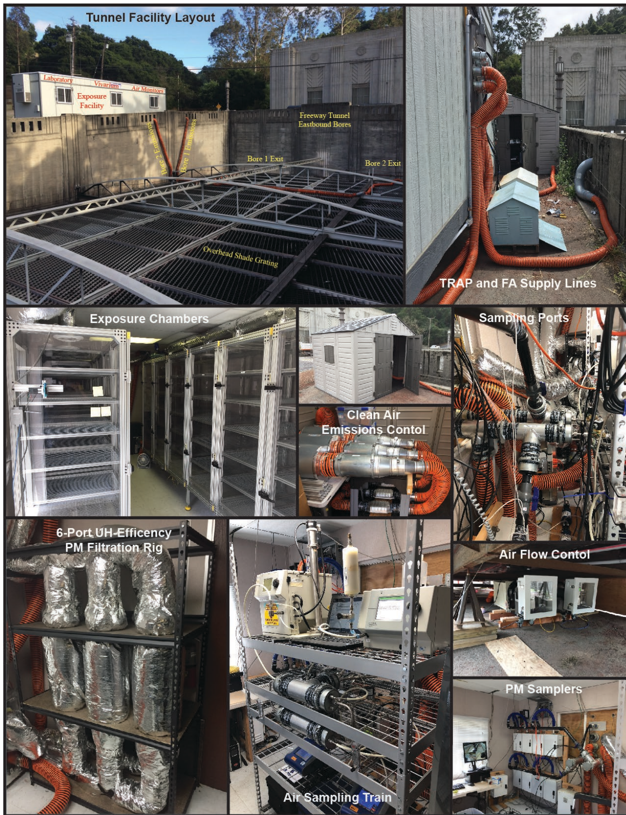
Figure S1. Photo montage of the various systems comprising the Tunnel Exposure Facility.
