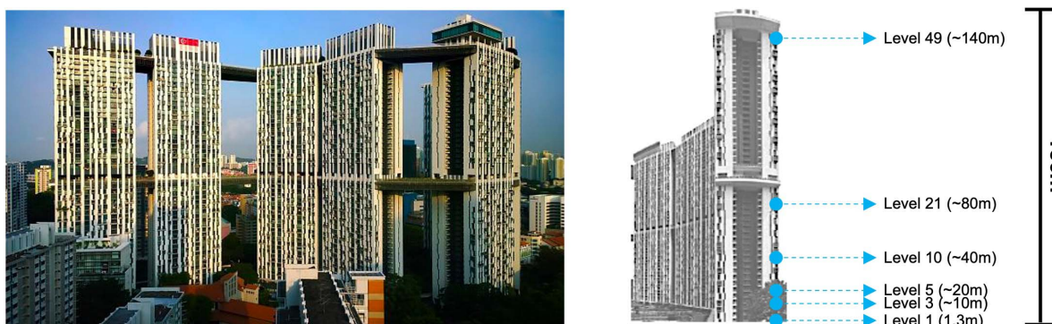
Figure S70. Vertical air sampling in the built environment. Overview of the sampling location at the Pinnacle@Duxton.
