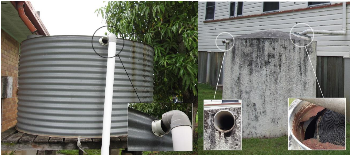
308 Figure 3. Non-compliant rainwater tanks (with anti-mosquito regulations) identified in Gin Gin containing Aedes aegypti .
