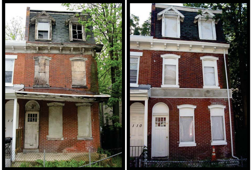
Figure. Abandoned housing remediation in Philadelphia.
