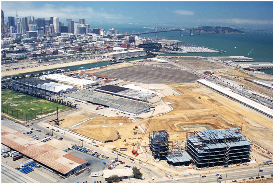
Figure 4. Genentech Hall under construction in Mission Bay. Image courtesy of UCSF.
