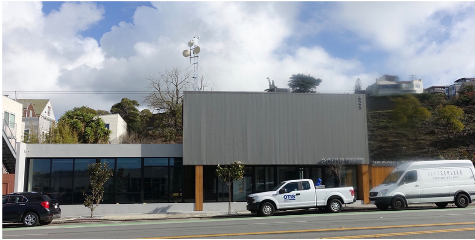
Figure 8. The new fixtures store that has moved into New Gen’s old building. Photo credit: the authors.
