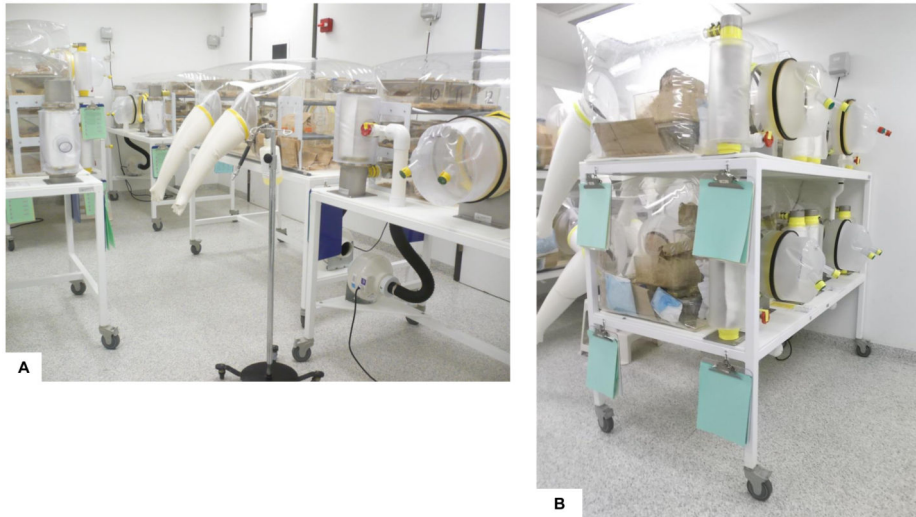
Figure 1. Flexible film isolator housing areas of the Gnotobiotic Research Animal Facility A. Single level tables with single large isolators. B. Double level tables with four isolators.
